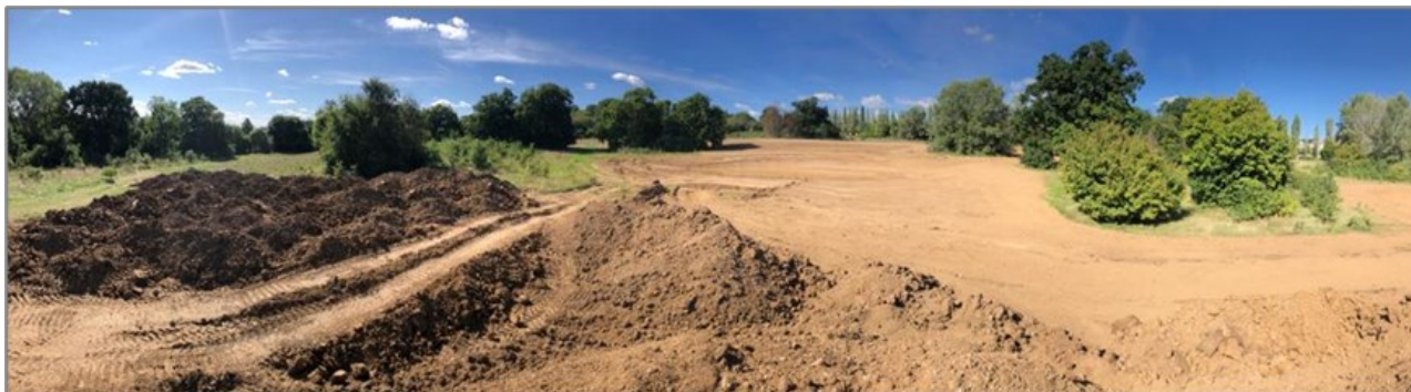
Photo: after the earth moving
