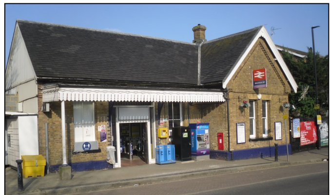
Winchmore Hill Station in 2021
