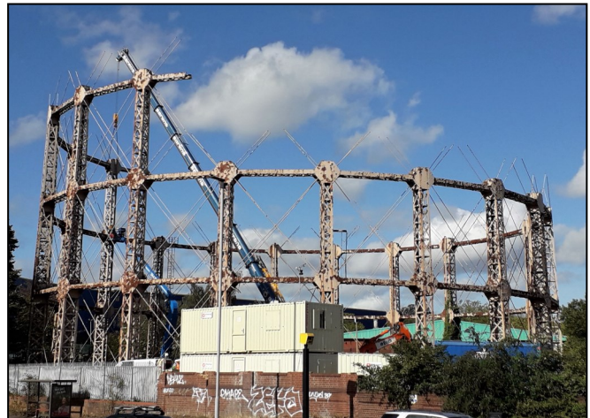
Dismantling the frame
