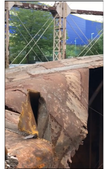
Partially cut up dome
