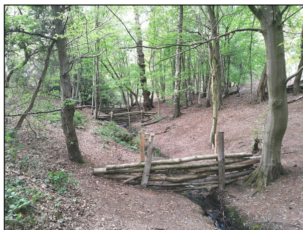
A typical “Leaky Dam” to reduce the risk of flooding
